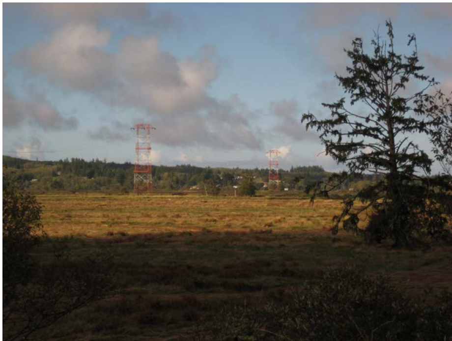
230-kv crossing of Youngs River
