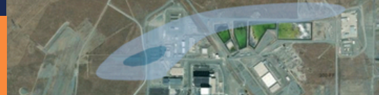
Tritium plume, showing high concentrations under 618-11
